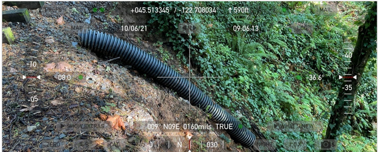
Exhibit 5-3: Replacement pipe installed at culvert 6
