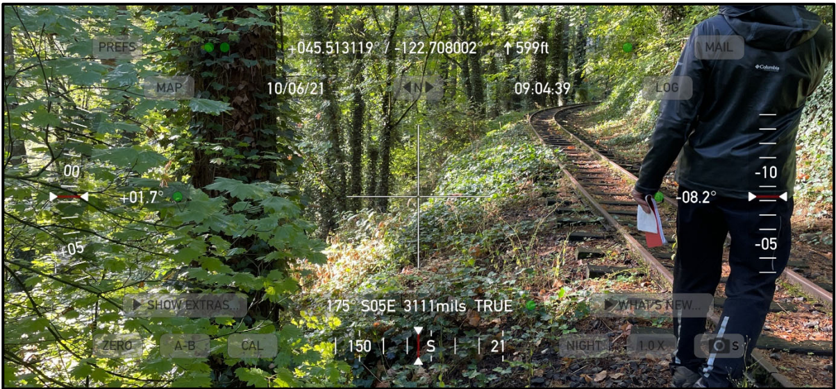
Photo TH000007: Crib Wall 2 / "Texas" Gulch looking south
