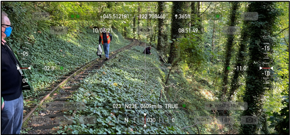
Photo TH000006: Potential slump west of tracks looking north
