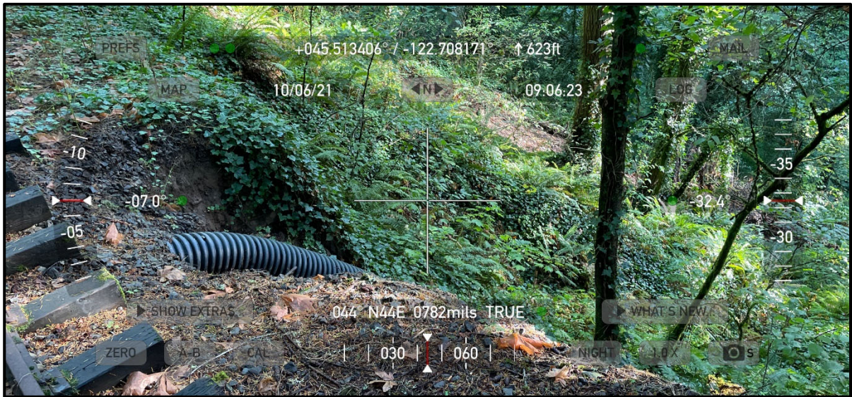
Photo TH000009: Culvert 6 looking north
