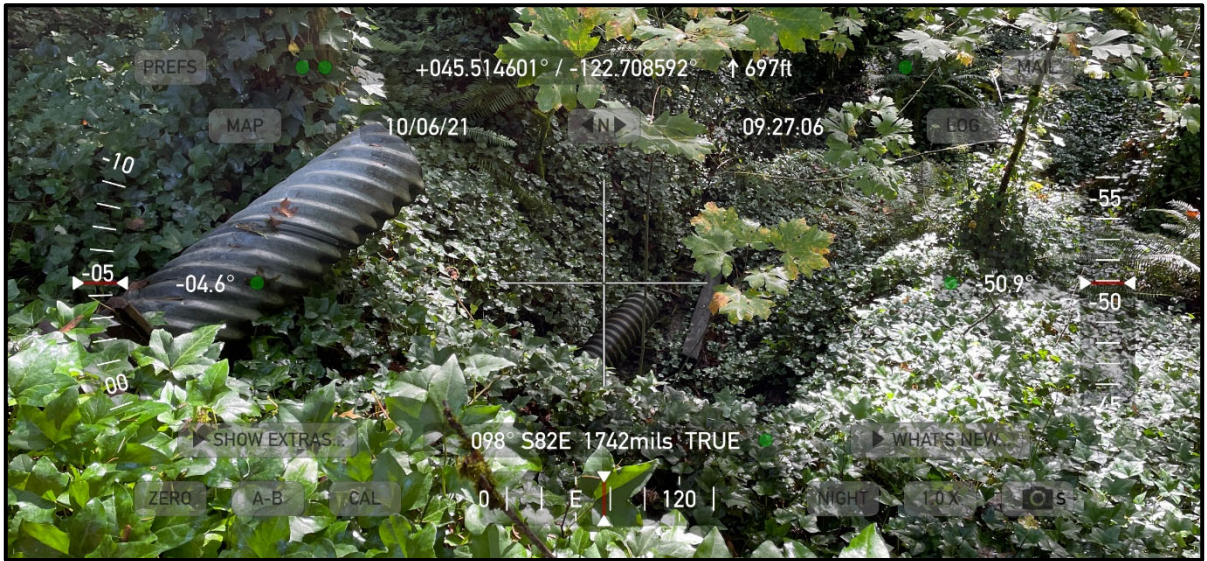
Photo TH000016: Culvert 8 looking southeast
