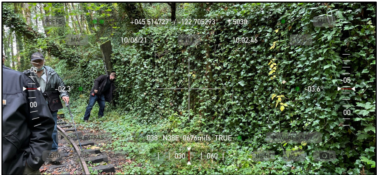
Photo TH00024: Timber Wall east of tracks near Culvert 14 looking northeast
