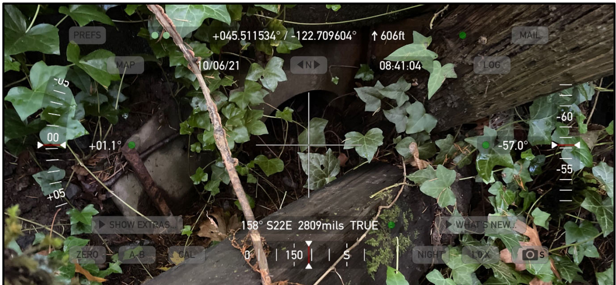
Photo TH000004: Culvert 3
