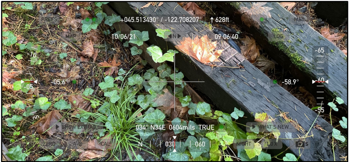
Photo TH00010: Culvert 6 underlying wood timbers
